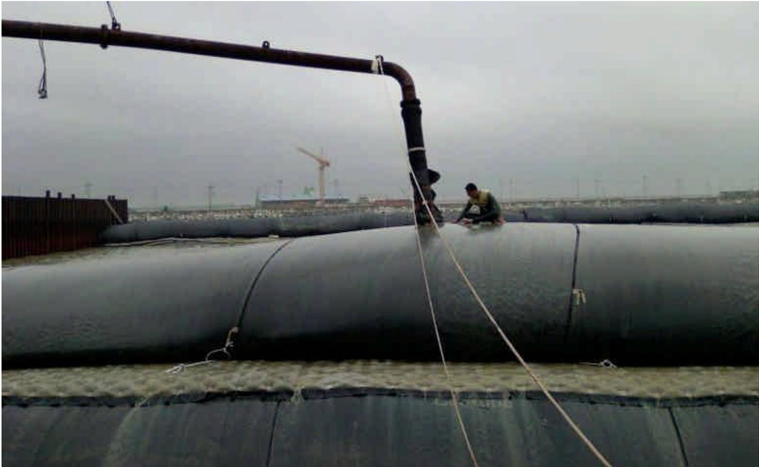
Pumping of 2<sup>nd</sup> level Geotube<sup>®</sup> with sand slurry
