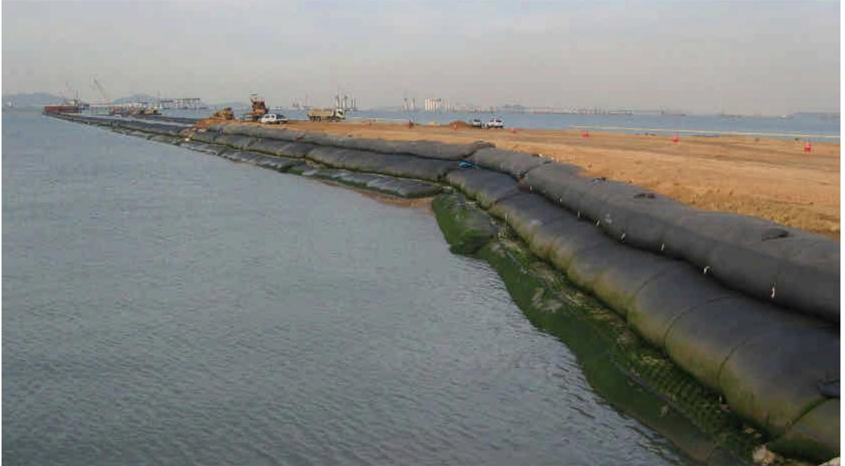
View of partially completed Geotube® artificial island
