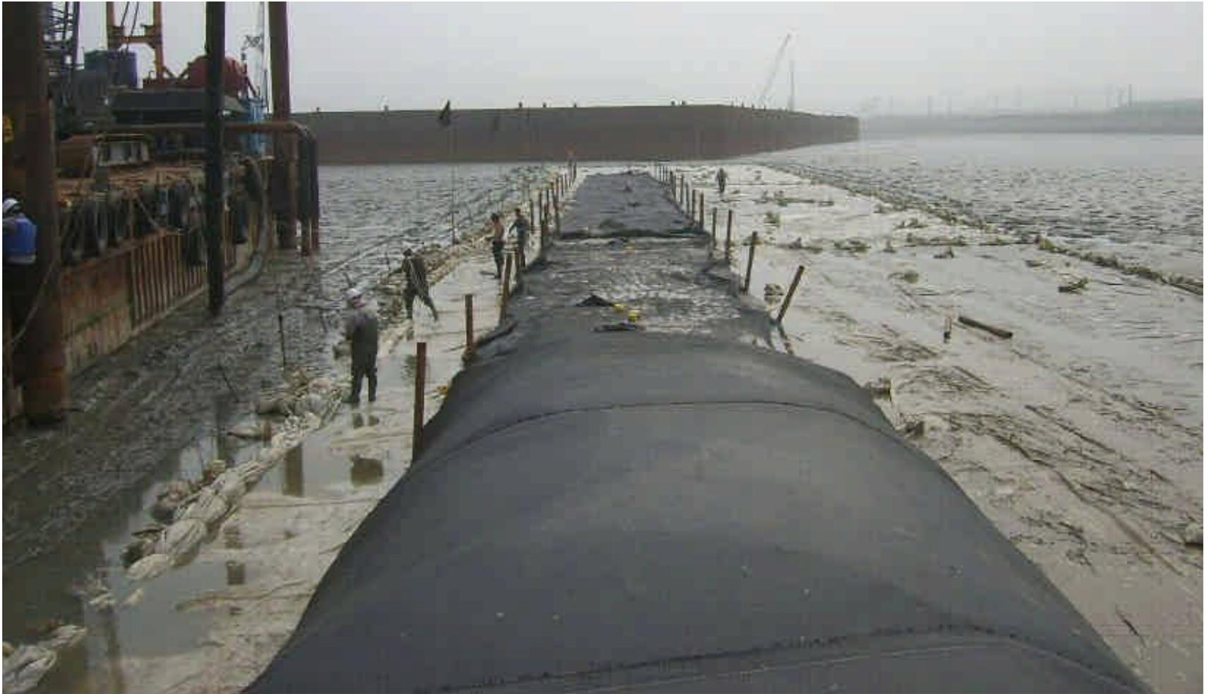
Laying of bottom Geotube<sup>®</sup> (outer) during low tide
