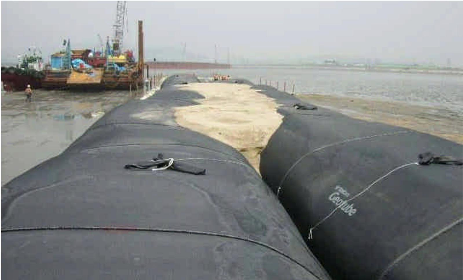
Sand filling and leveling between bottom Geotube<sup>®</sup> systems during low tide
