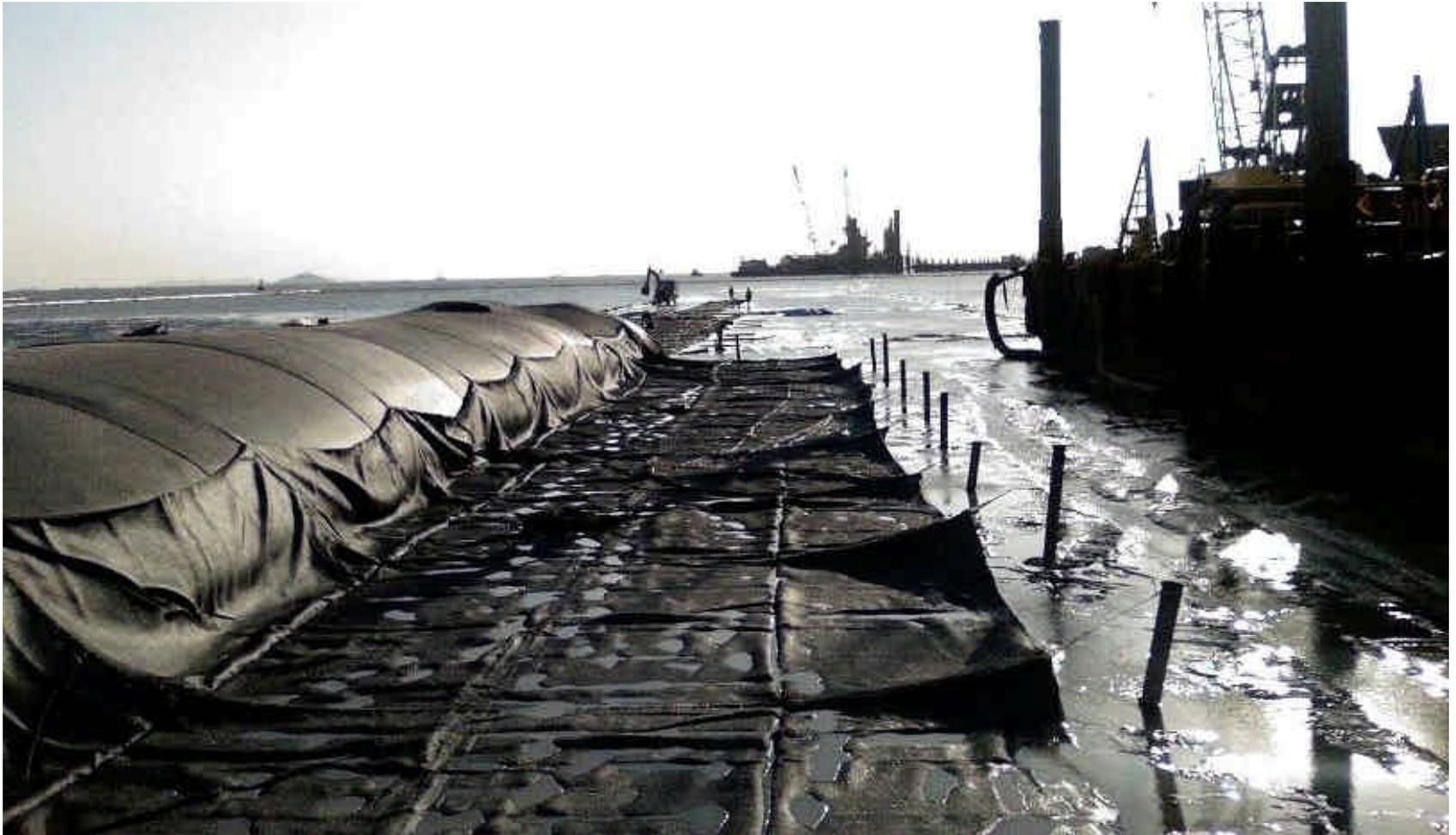
Laying of bottom Geotube® (inner) during low tide
