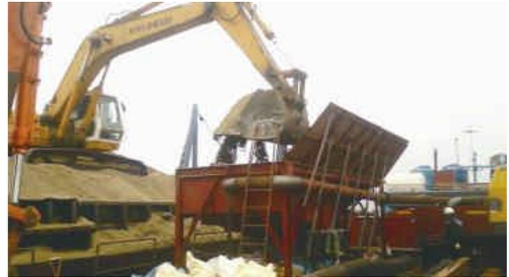
Placing sand into slurry mixing tank
