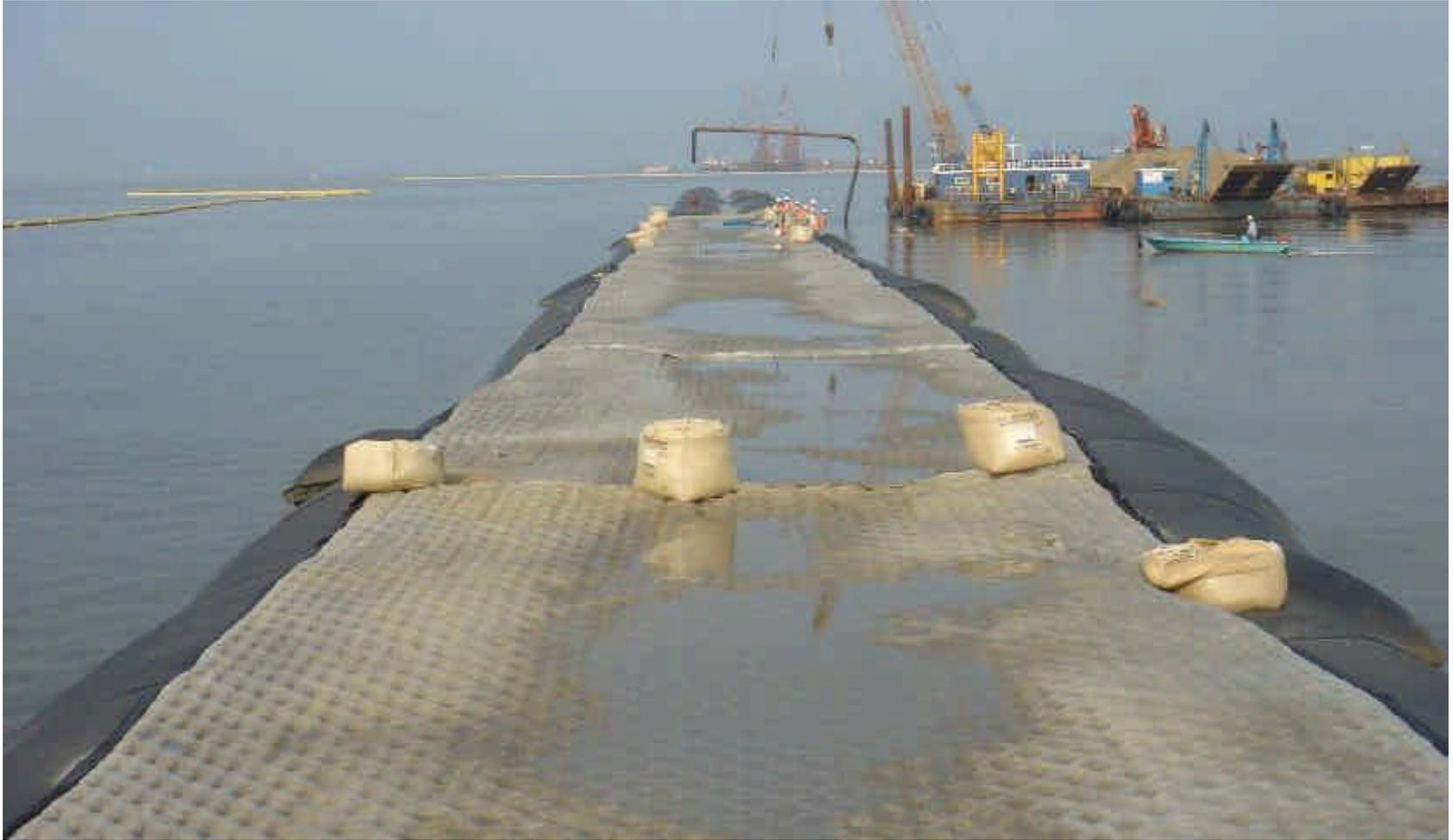
Installation of sand mat above bottom Geotube® systems
