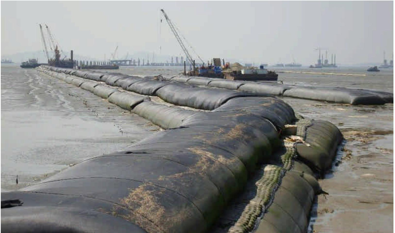
**Bottom & 2<sup>nd</sup> level Geotube<sup>®</sup> completed for 1 side of artificial island**
