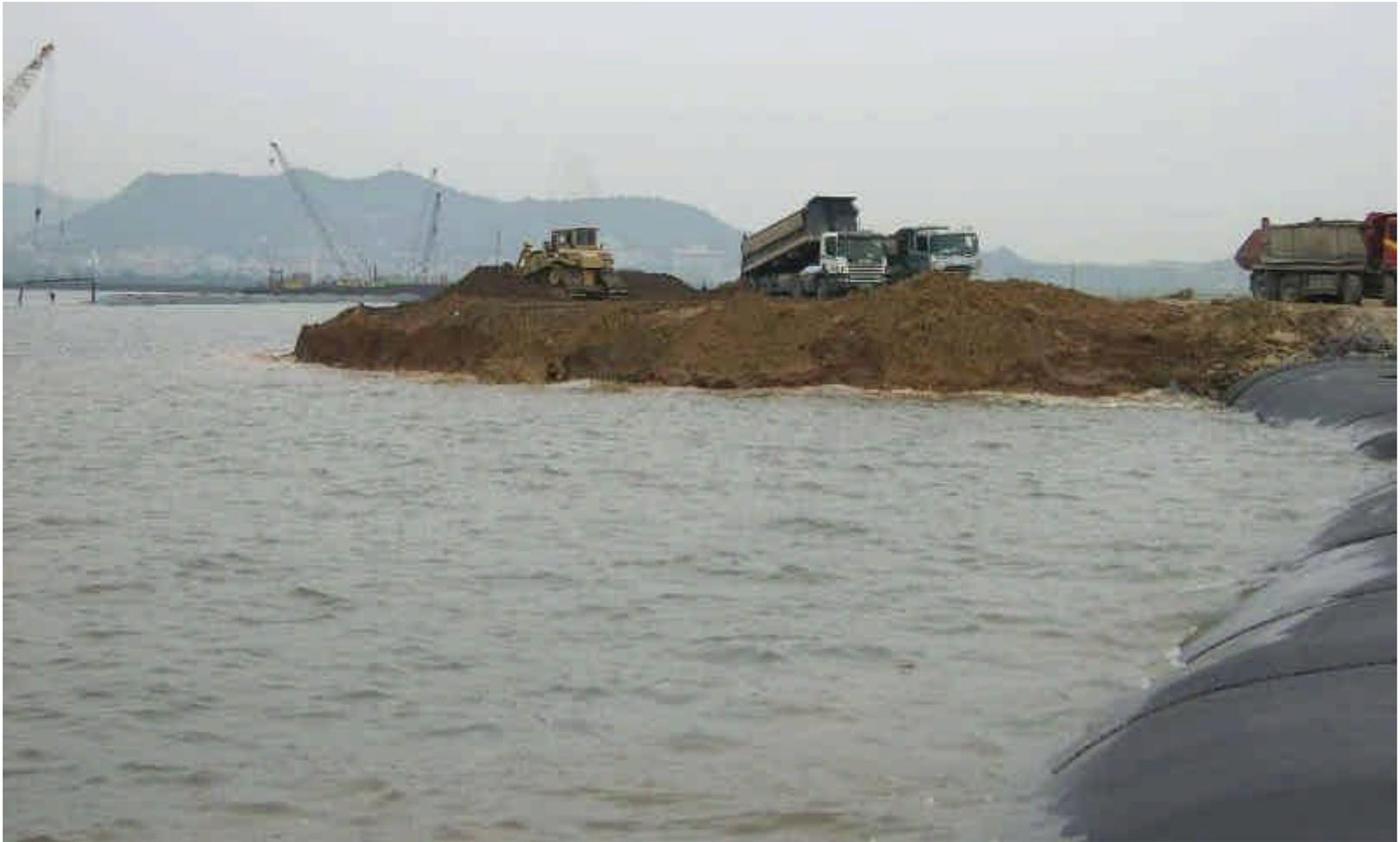
Backfilling behind Geotube<sup>®</sup> dyke with residual soil
